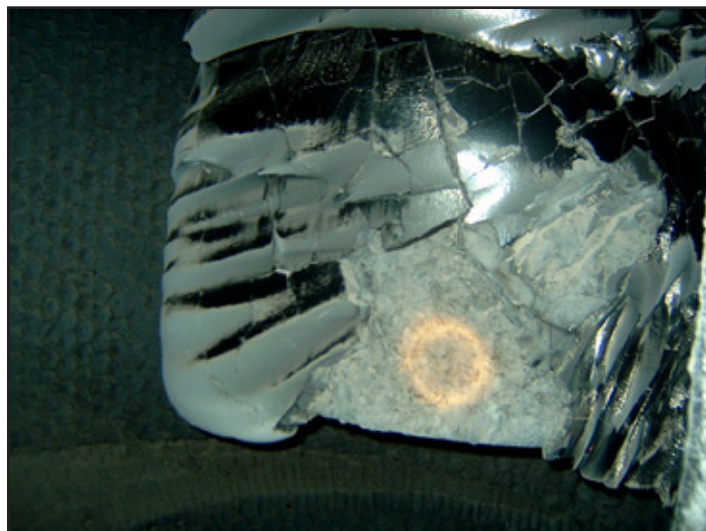
Figure 1: Coke deposit on outer portion of reactor cyclone vapor tube. Note area of coke spalling.
