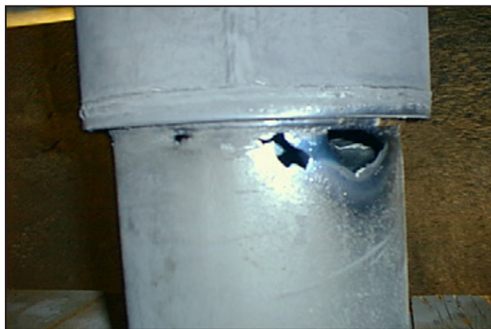
Figure 2: Picture of erosion in cyclone dipleg.
