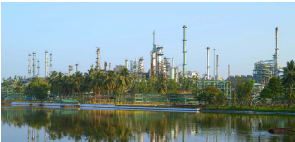
Figure 1. The BP Kochi refinery recently expanded its risk based inspection (RBI) process. Photo courtesy of Meridium, Inc.
