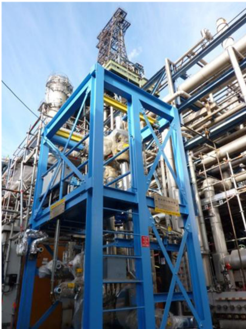
Figure 1. Industrial Scale Test Filter at a Refining Facility for Online Testing.
